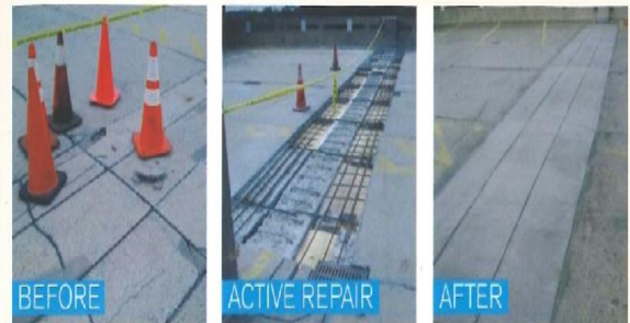
Photos of ASD -Repairs
