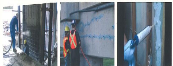
Repair by shotcrete
