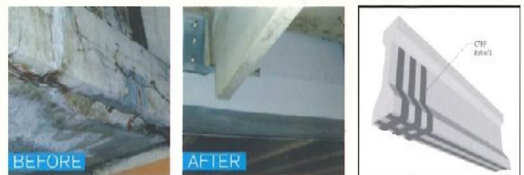
Photos of ASD -Repairs
