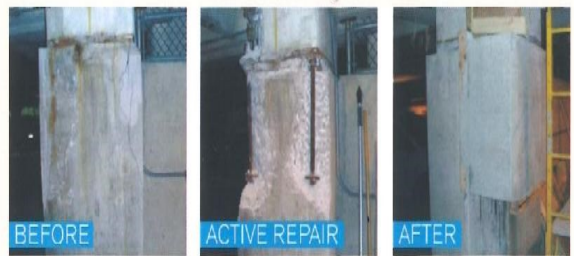
Photos of ASD -Repairs
